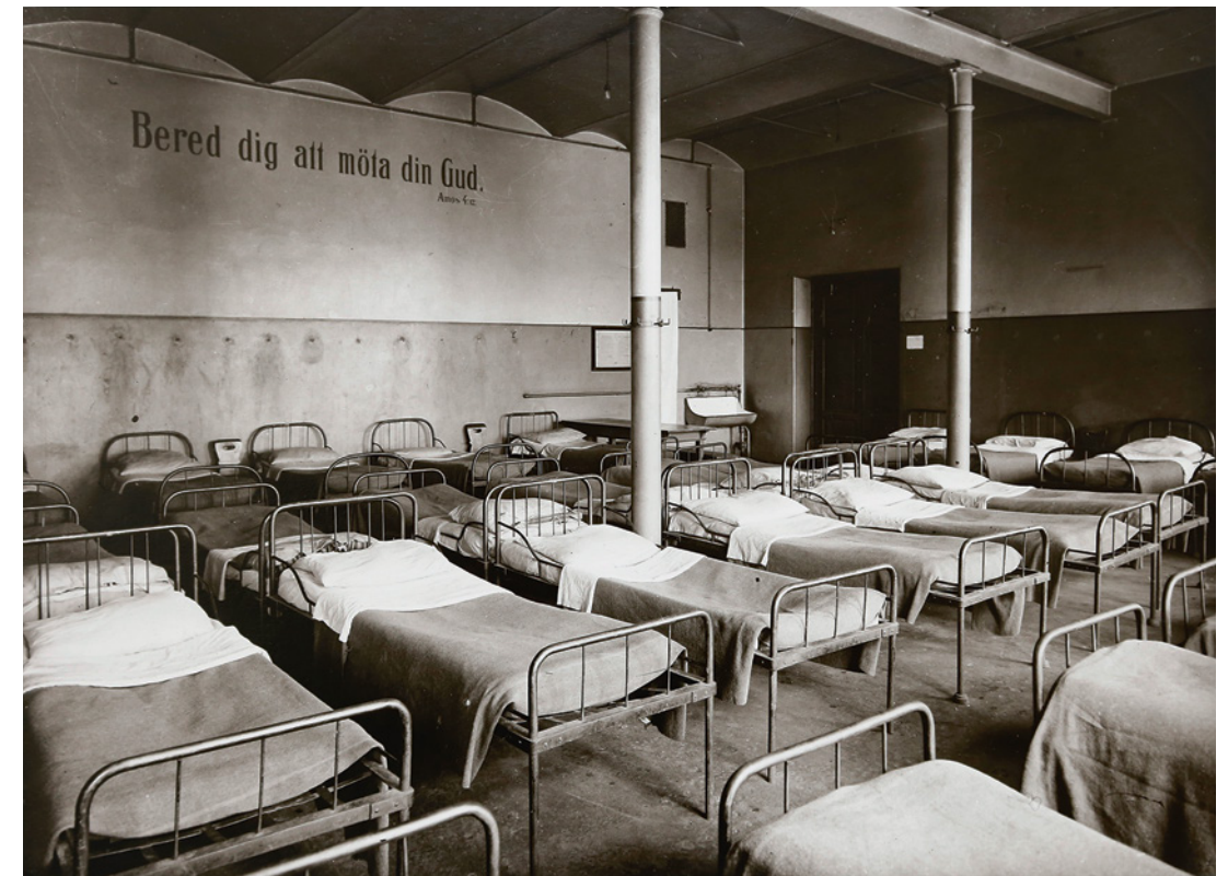
“Prepare to meet your God,” painted on the wall of Pursimiehenkatu 10 shelter in Helsinki in the 1920s.
